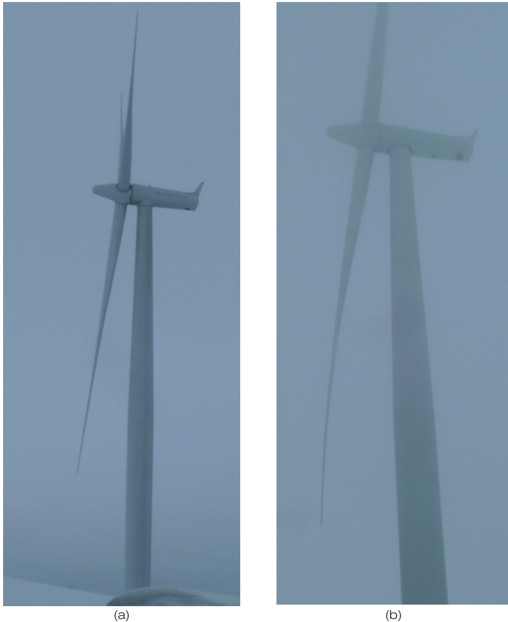
Figure 3: Wind turbine blades: (a) under no wind condition, (b) blades are moving and producing power [7]
